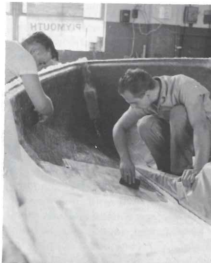
Laying up an early hull at the first Oakland, MD plant.
