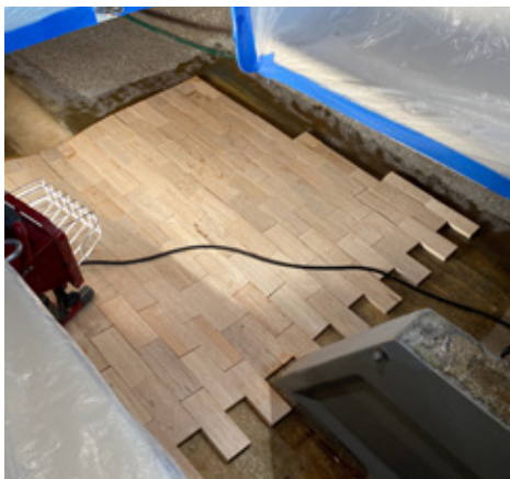
Balsa in place aft.
