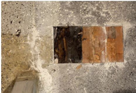
Assessing the damage.
