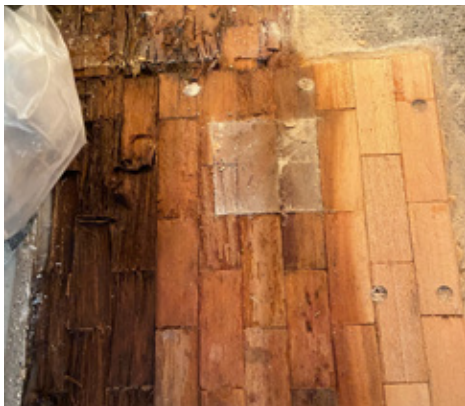
The entire core was wet.
