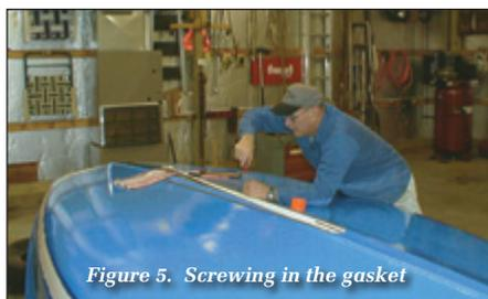
Figure 5. Screwing in the gasket
